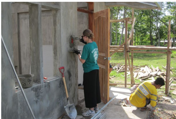
Volunteer completing simple masonry work
