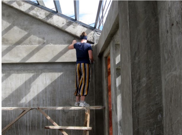
A volunteer scrapes the walls to clear the wall surface
