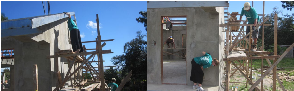
Volunteer scrapes the walls outside the building
